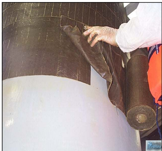
◀ Figure 4. Marine Piling Tape overlap of roll ends.
