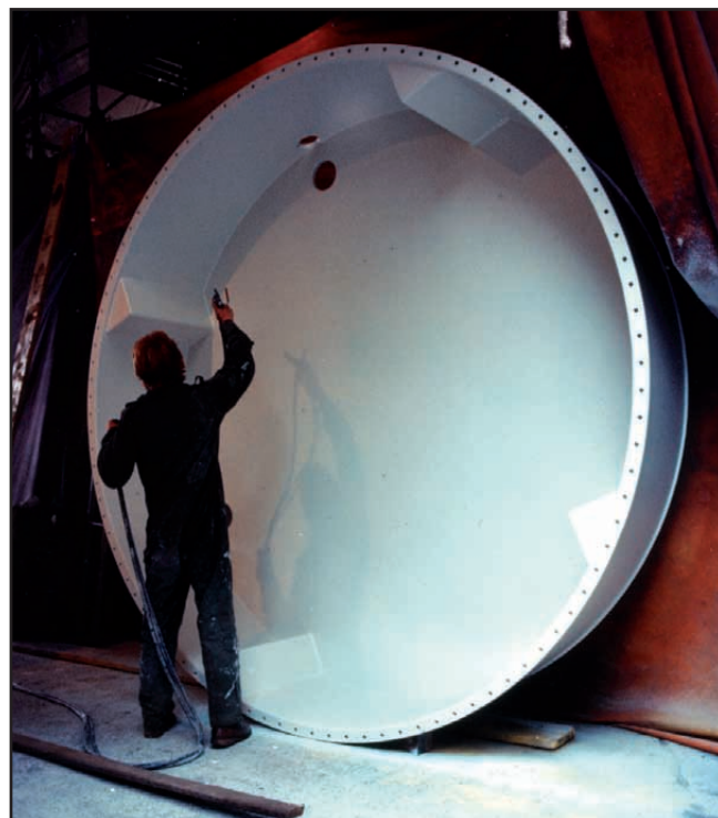
Application of 400 Series glass flake lining to mild steel process vessel.
