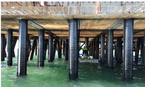
HP2 Octagonal Steel Piles protected with Denso SeaShield 2000FD Series
