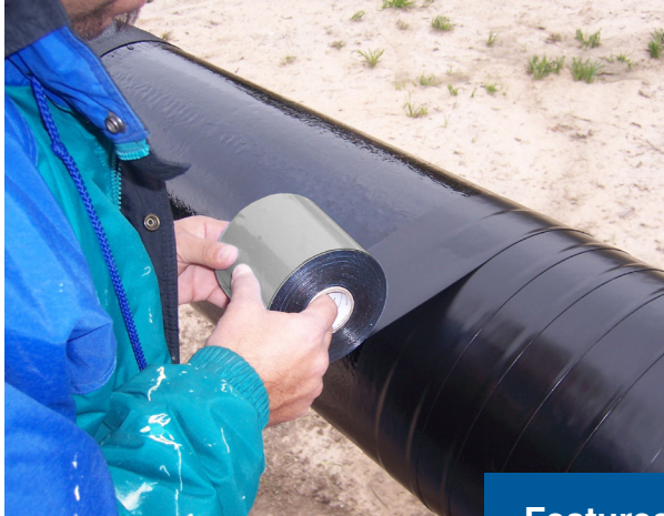
Application of Denso Butyl Tape.
