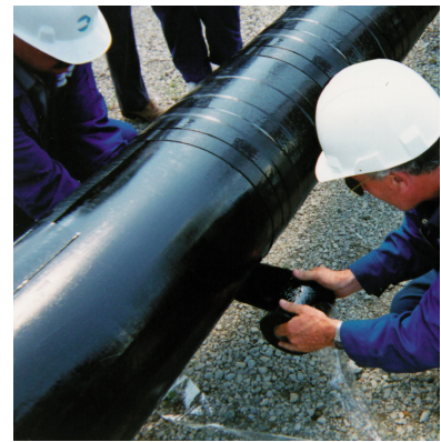
Application of Densopol 60 Tape.
