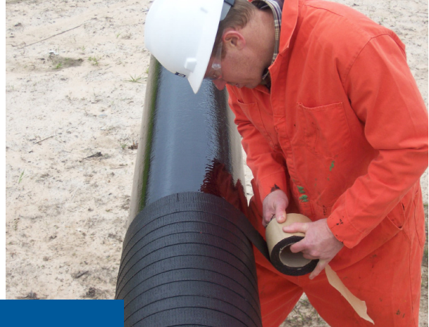
Application of Denso MB-50 Tape.
