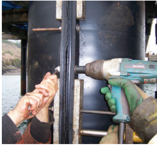
The SeaShield™ Series 2000FD System features a controlled application tensioning system.
