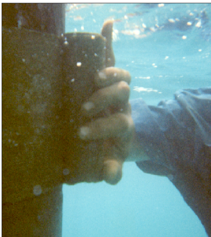
▲ Figure 3. Tape being applied under water.
