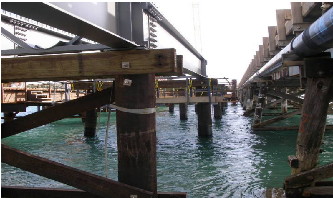
► Figure 2. Timber piles protected in the splash zone.
