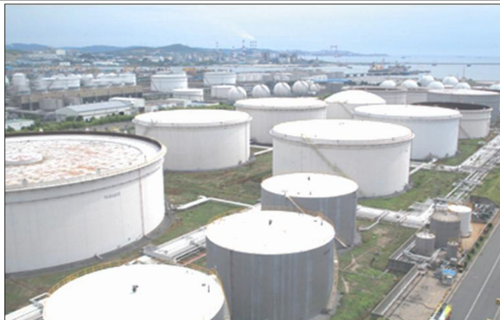
▲ Figure 1. Tank farm.
