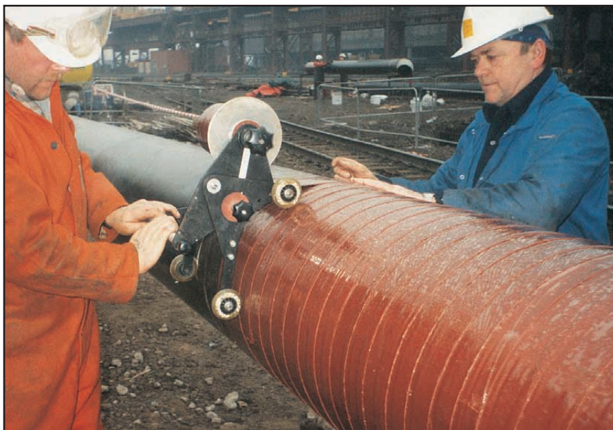
Fast Densoman Machine application of Denso Hotline Tape.
