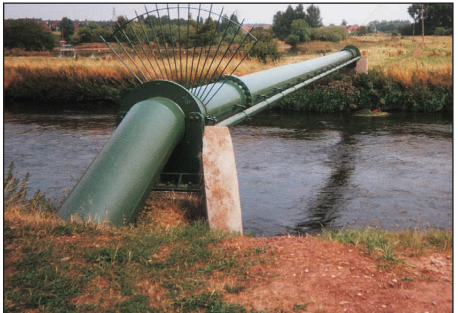
Below: Steelcoat 700 System protecting a pipebridge.
