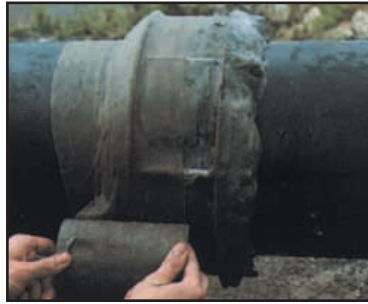
Overwrapping with Denso Tape
