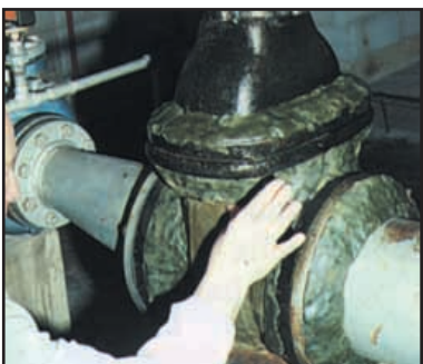
Profiling with Densyl Mastic.
