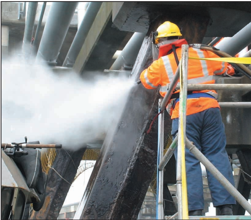
High pressure water-jetting.
