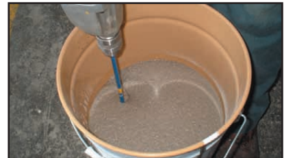
Mixing the 550 Epoxy Grout.
