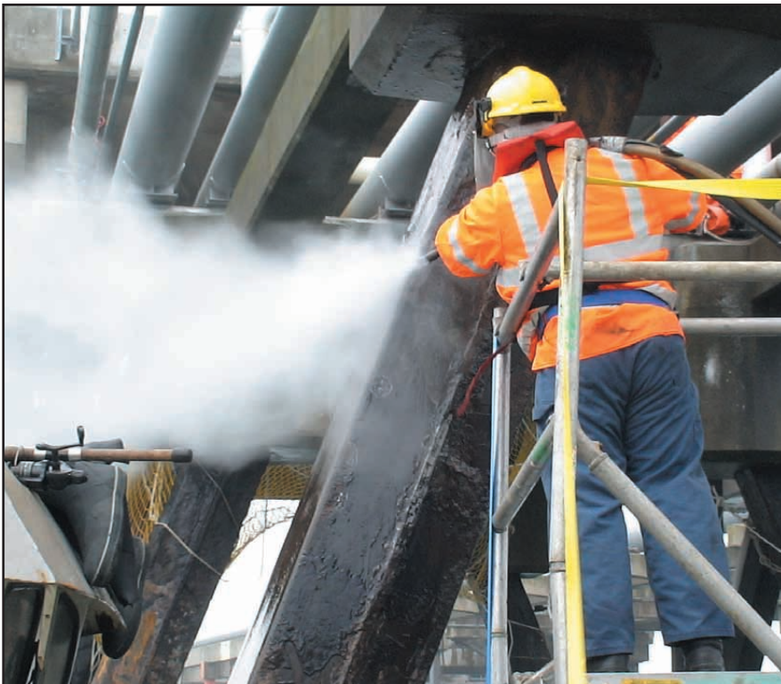
High pressure water-jetting.
