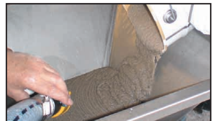
Pouring the Grout into the pump hopper.
