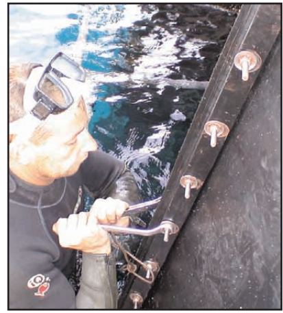
3. Final tightening of the 316 stainless steel bolts.
