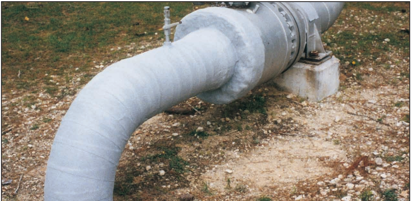
Above: Application of Denso ColourTape Mastic - no primer necessary. Below: First section of exposed pipe and flange fully coated with the Steelcoat 300 System.
