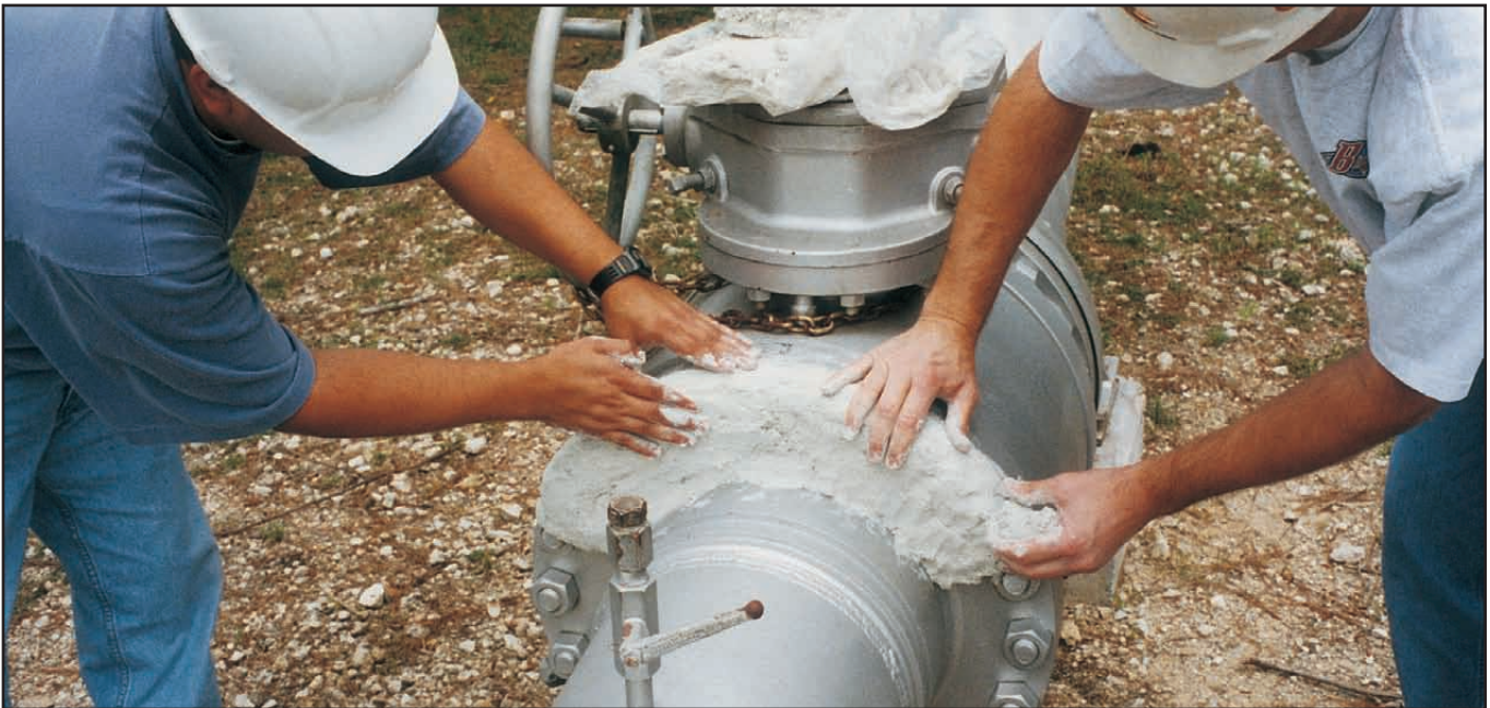
Above: Application of Denso ColourTape Mastic - no primer necessary. Below: First section of exposed pipe and flange fully coated with the Steelcoat 300 System.
