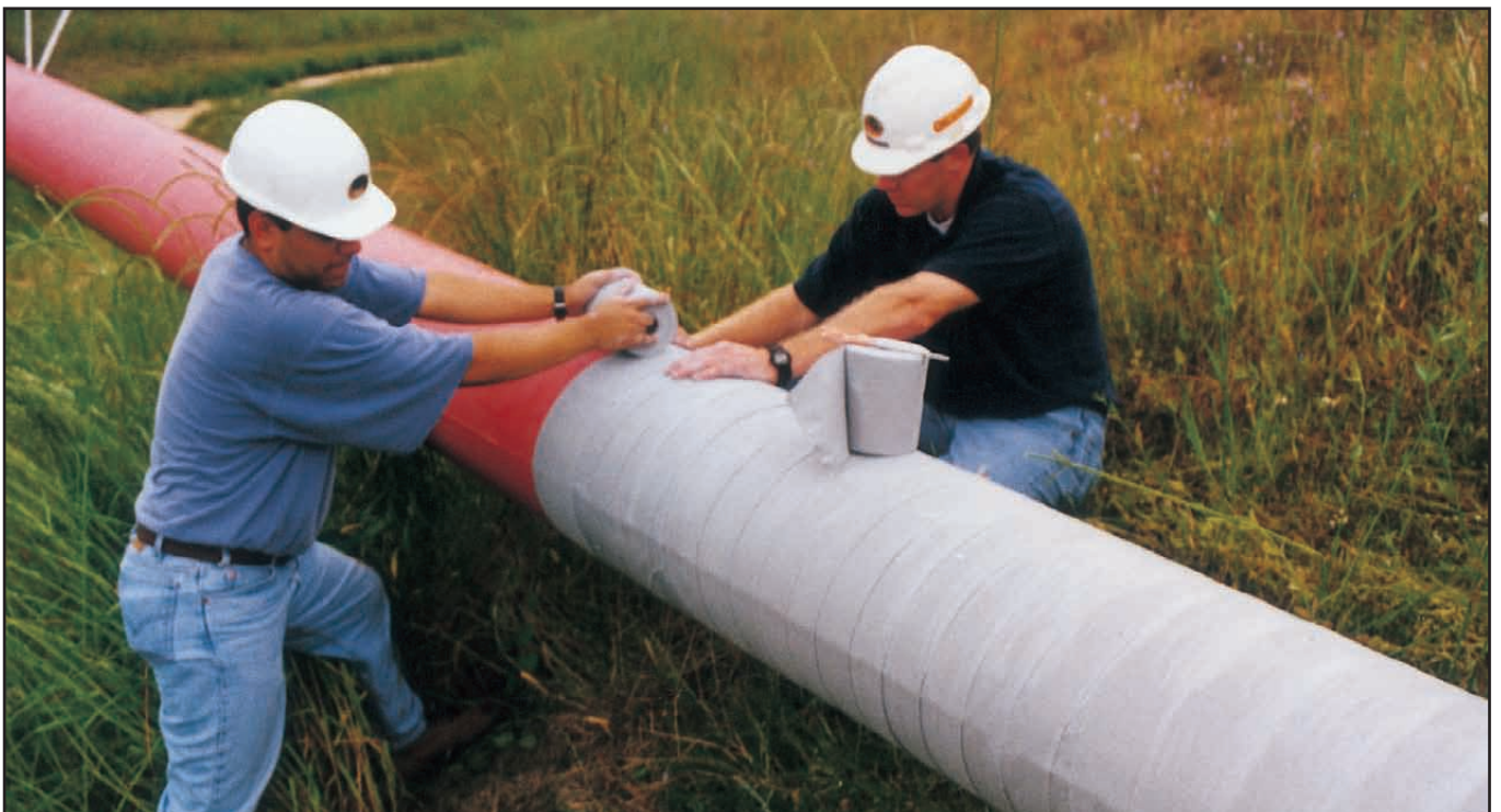
Fast hand application of Denso ColourTape.
