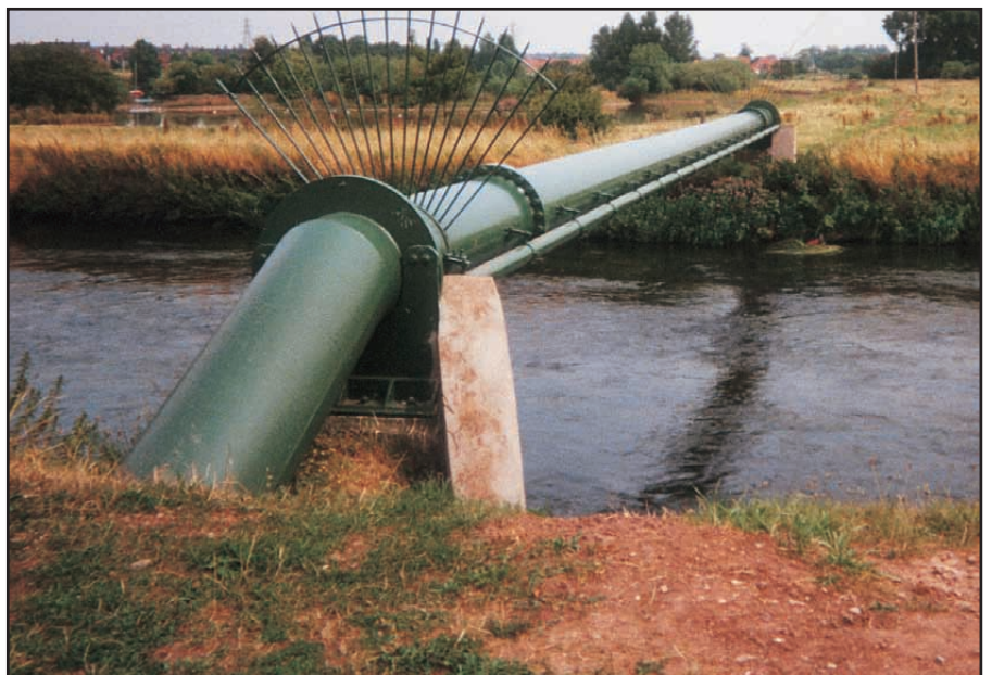
Below: Steelcoat 700 System protecting a pipebridge.
