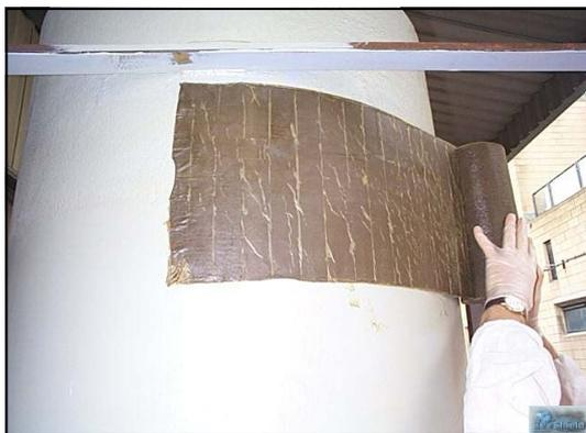
In the pile protection zone apply the tape by starting with two full circumferential wraps then proceed spirally along the pile progressing with a 55% overlap, giving effectively a double layer of tape. This will ensure a minimum double thickness of tape all the way. Carry on until the roll runs out. Commence each new roll by overlapping the last roll by the same length as the tape width, for example if the tape is 150mm wide then the overlap will be about 150mm.
