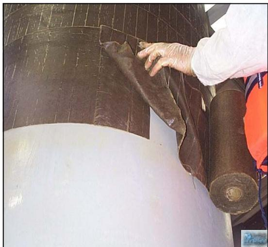
It may be worthwhile assessing the number of jackets that can be applied and the tidal conditions so that only enough tape is applied for the same number of jackets that can be fitted in a day. The tape that is then left exposed should be temporarily protected with some spare HDPE sheet until the job can be finished. Do not leave tape only exposed to the elements and the sea as it may become dislodged before the job can be completed and will have to be discarded and the piles rewrapped.
