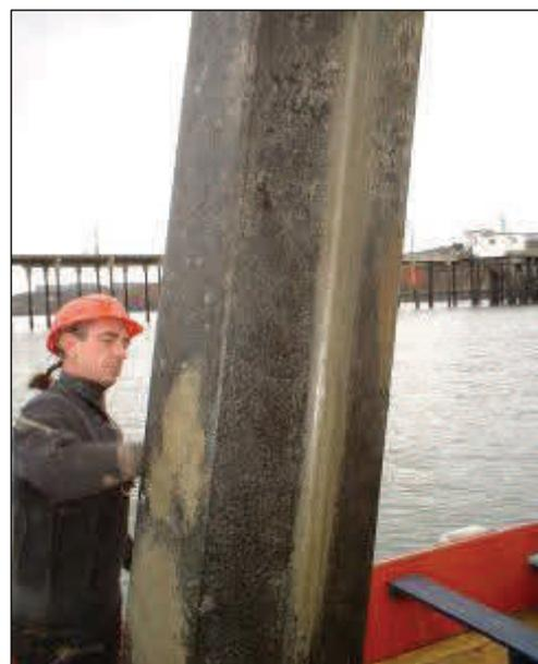
**Figure 2.** Cleaned pile showing the application of primer down the sides of a vertical weld seam and into pits. Shown is a hexagonal steel pile. The procedure is the same for circular concrete or
