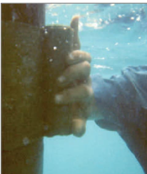
▲ **Figure 3.** Tape being applied under water.
