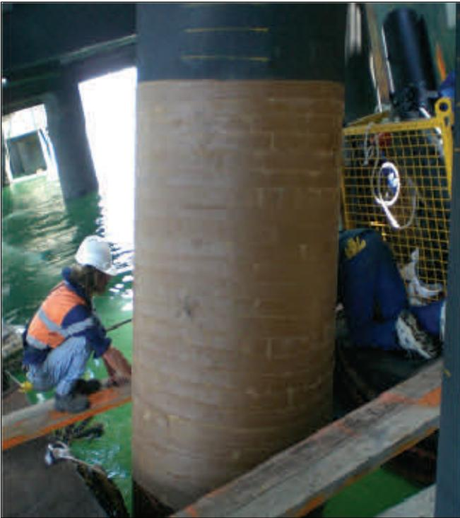
As wrapping proceeds smooth by gloved hand to exclude water, air bubbles and wrinkles from under the tape and to aid sealing of overlaps. Any overlapped edges are to be moulded and blended together by hand. This process is repeated all the way along the protection zone finishing again with two complete horizontal turns of the tape.
