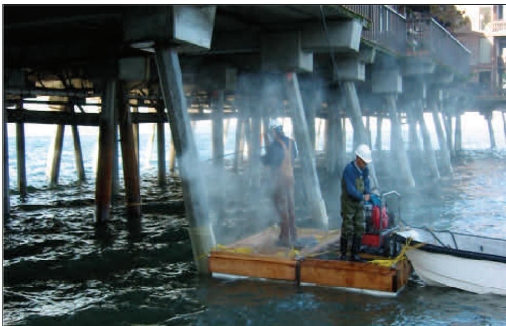
**Figure 1.** Preparing surface with high pressure water blasting. ▲
