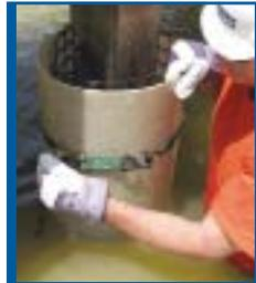
Marine timber piles are susceptible to damage while in service. Conventional repairs involve a fiberglass jacket that is filled with steel reinforced cementitious grout. Since normal reinforcing steel is often used, adequate cover of the steel bars must be maintained. This results in a large gap between the fiberglass jacket and pile resulting
