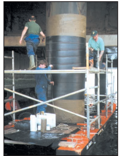
Installation, Coal Jetty, Scotland.
