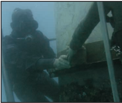
Underwater tape application, Australia.
