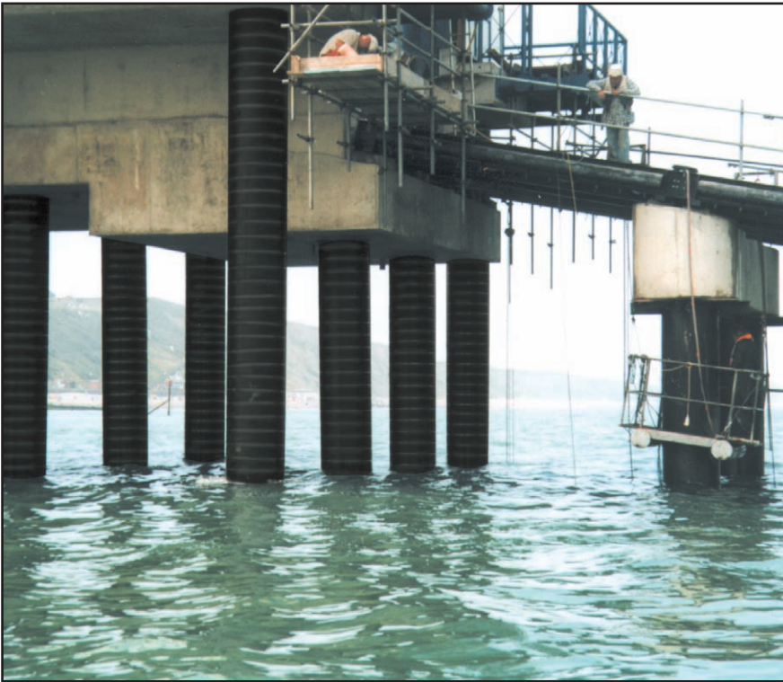
New lifeboat slipway, Cromer UK.
