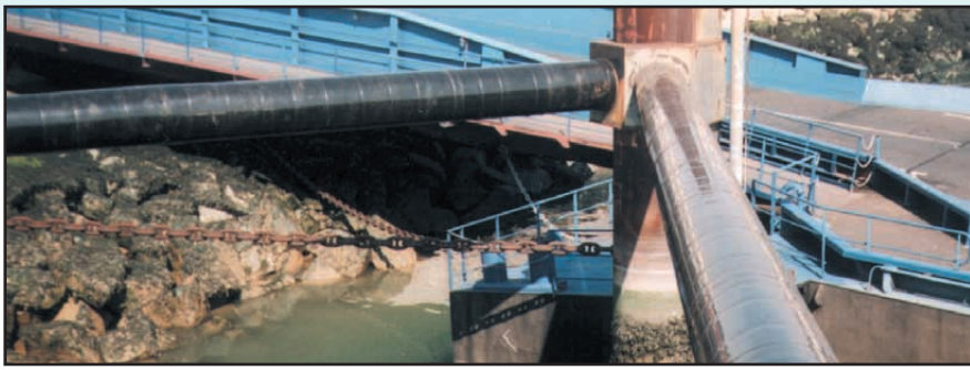
Pile bracings Ro-Ro berth, Ramsgate, UK.
