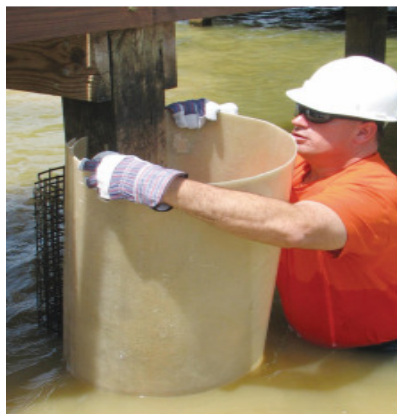
Figure 3. ▲ SeaShield Fiberglass Jacket is then snapped in place around the C-Grid ® 450
