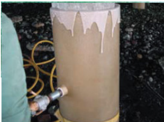
Figure 6.> SeaShield 550 Epoxy Grout pumped into the annulus around an existing octagonal concrete pile
