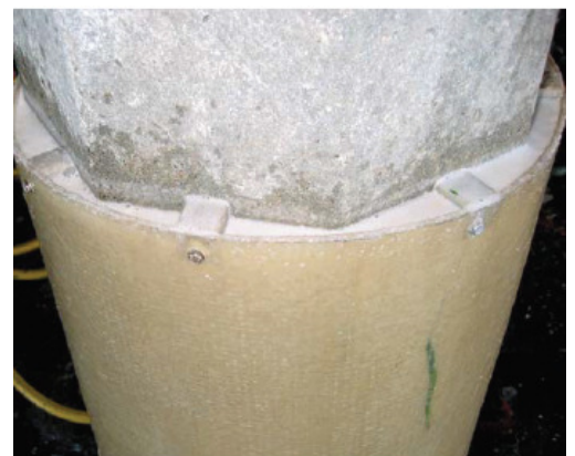
Figure 5.< SeaShield 550 Epoxy Grout being pumped into the SeaShield Series 500 Fiber-Form
