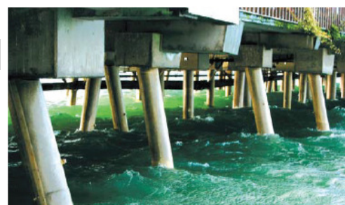
Figure 1. & 2. > Marine piles protected by Denso SeaShield Series 500 System
