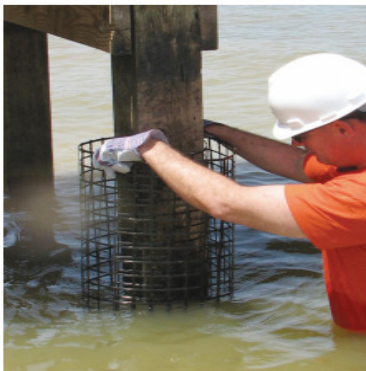
Figure 2. Lightweight and non corrosive C-Grid ® 450 is installed around the pipe
