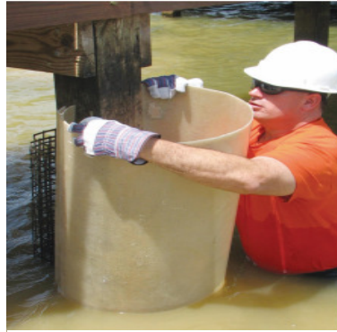
Figure 3. SeaShield Fiberglass Jacket is then snapped in place around the C-Grid ® 450
