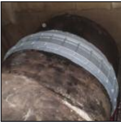
Application of paint primer.
