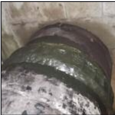
Application of Denso Mastic.
