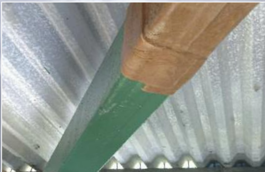
A Denso Petrolatum Tape system was used on steelwork in the conveyor tunnels
