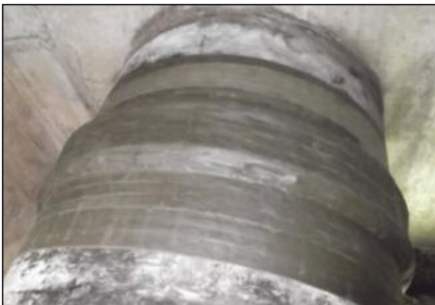
An overwrap of Denso Tape completes the protection.
