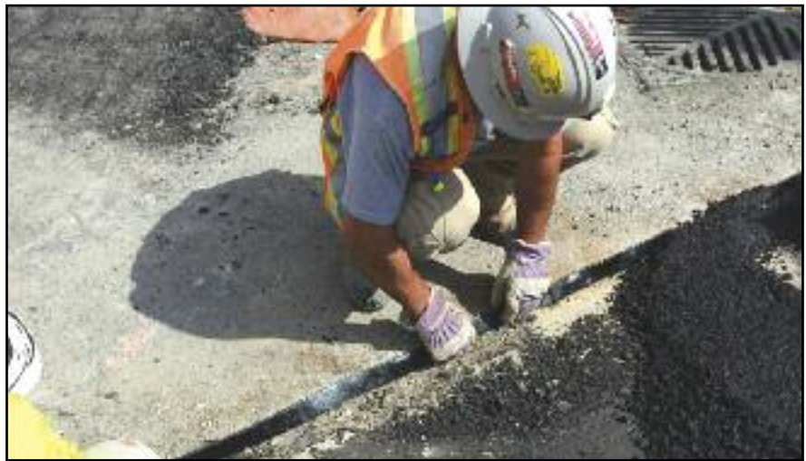
Densoband is applied to the vertical joint face of the reinstatement trench providing a waterproof and flexible seal over the entire depth of the joint.
