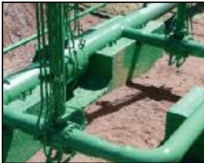
Pictures: All steel parts of the valve stations were protected with Protal 7200.
