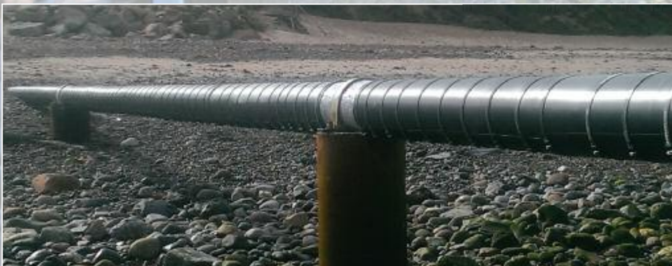
Above: Damage to the cement mortar on the Jurby outfall pipe.
