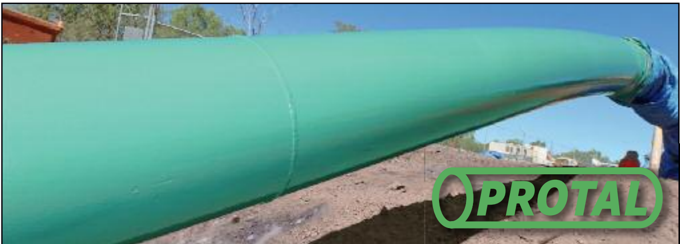
Pictures: All steel parts of the valve stations were protected with Protal 7200.
