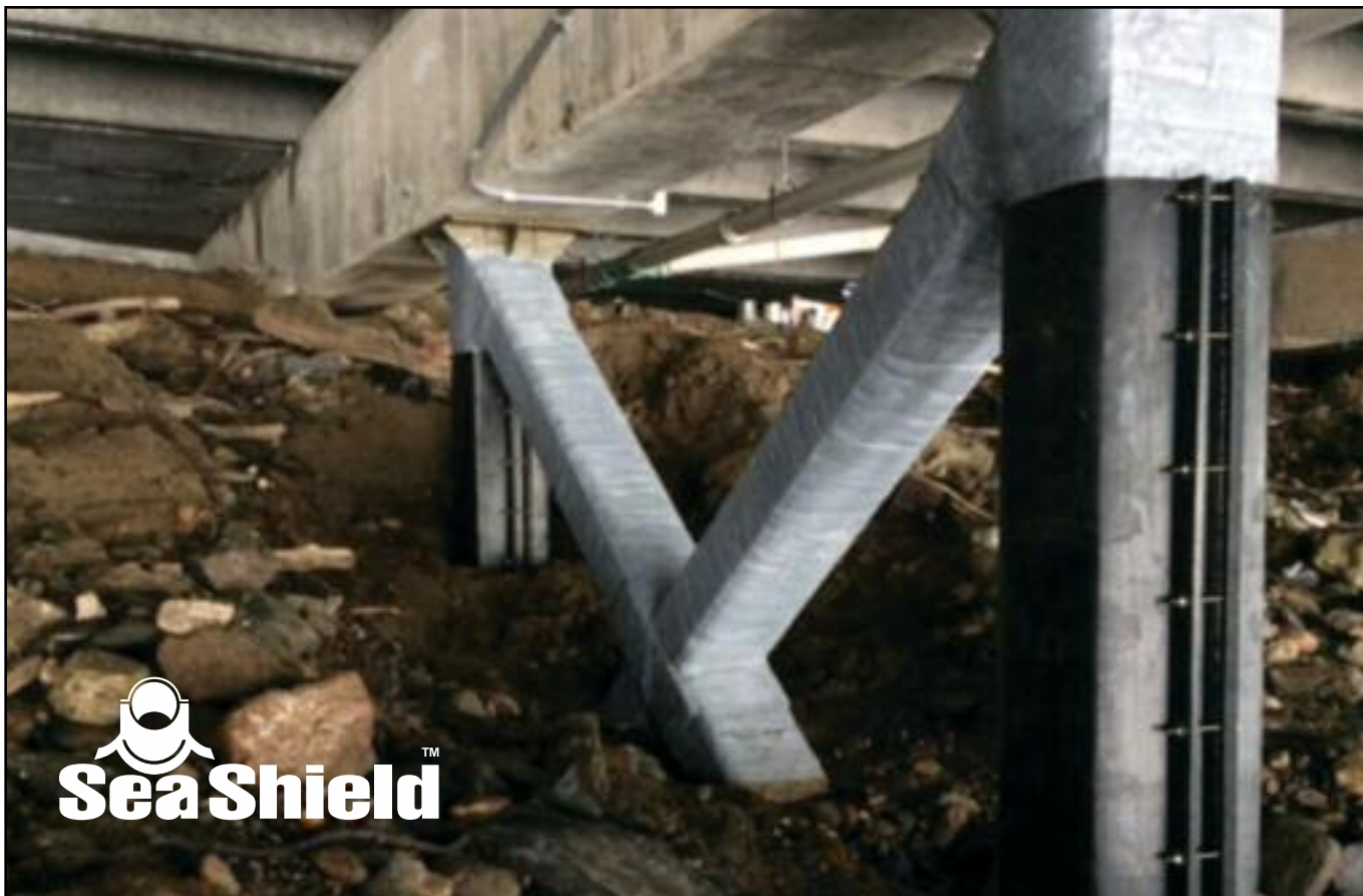
Above: Pile cap/gusset area protected with the SeaShield SplashZone UW Epoxy.
