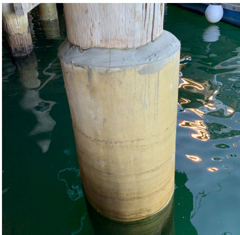
The Denso SeaShield Series 70™ and SeaShield Series 400™ Systems as used on the Appleton Dock Wharf refurbishment.
