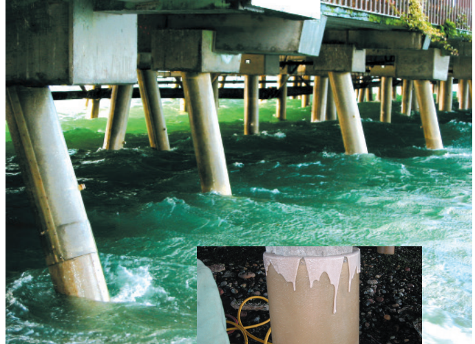
SeaShield™ 550 Epoxy Grout being pumped into the SeaShield™ Series 500 Fiber-Form Jacket.
