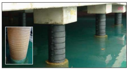
Wharf 14 showing installed Seashield Series 100 system. Inset shows the Denso Marine Piling Tape that forms the heart of the system underneath each jacket.
