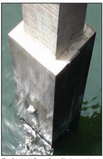
The Seashield Epoxy Grout fills the annulus between the pile and the SeaShield Jacket.
