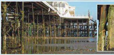
Above: Worthing Pier, Sussex - inset shows heavy marine growth cleaned off of a SeaShield jacket revealing it to be in good condition underneath and perfect working order after 27 years in service
