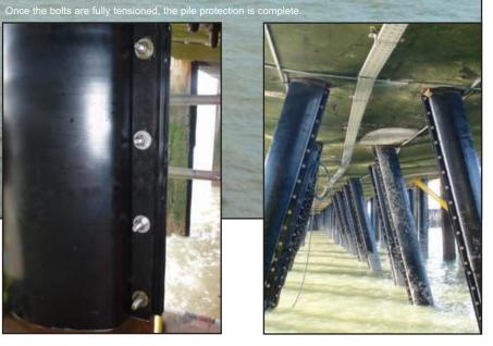
A Denso SeaShield system was again chosen to protect the new independent fender piles as well as the existing piles from the corrosive marine environment. This can be a major problem in splash zones, inter-tidal and subsea environments and the difficult area where the jetty pile meets the jetty platform.
