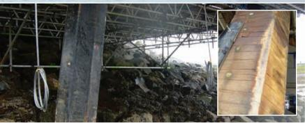
Above: The Kyle of Tongue Bridge in Scotland - inset shows close up of the excellent condition of the Denso Marine Piling Tape revealed upon jacket removal for inspection, after 22 years service.
