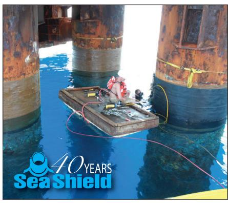
Securing the SeaShield 2000 FD outercover with the hydraulic tensioning tool
