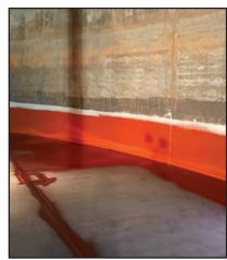
Archco 400 primer being applied to the blasted floor and side walls of the tank.
