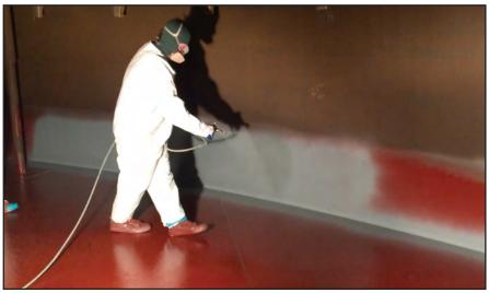
Archco 476P applied over the Archco 400 primer to provide excellent chemical and high temperature resistances.
