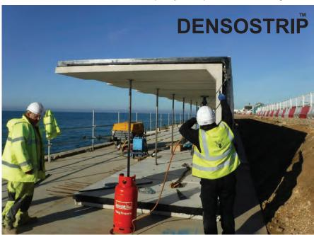
between joint faces previously primed with Densostrip primer. As well as water and sea water it is resistant to chemical and biological attack.
