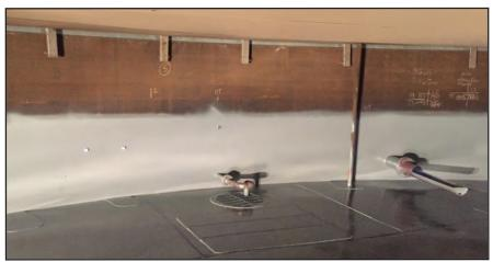
Fully cured Archco 476P lining providing corrosion protection and allowing the tank to return to service within 8 hours
