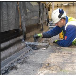
Above and below: After a single layer of Denso Ultraseal RT Tape is applied, a coat of Denso Topcoat completes the Steelcoat system application.
