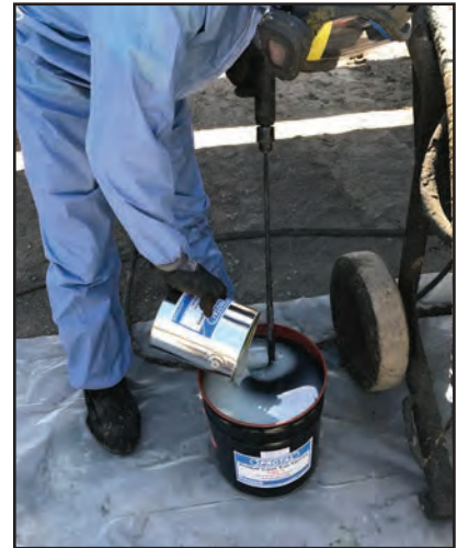
Protal 600 CTE™ Part "A" & "B" being mixed prior to the spray application.
