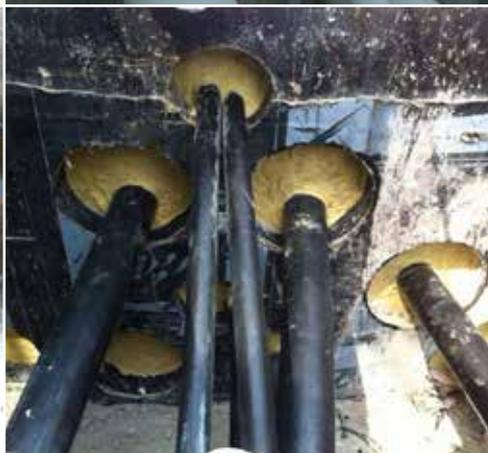
Densoseal 16A™ is a self supporting non-setting mastic which has been developed for sealing cable ducts and conduits against gas or water. It also has British Telecom type approval.
