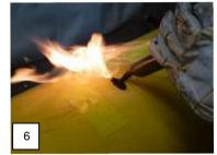
Continuously warm the repair stick and the area to be repaired.
