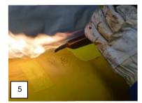
Preheat the repair stick with a flame until the material is soft. A light ignition of the repair stick is acceptable.
