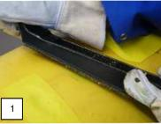
Remove any non-adherent factory coating and chamfer sharp edges with a rasp (semi-circular blade)
