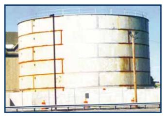
Above: Foremost area of Tank is treated with HoldTight 102. Flash rust is clearly visible either side of where the HoldTight was applied.
