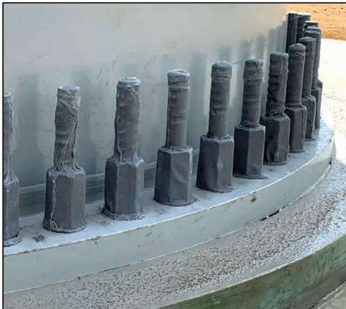
Denso™ ColorTape recently installed on 76 exterior anchor bolts on wind turbine tower
