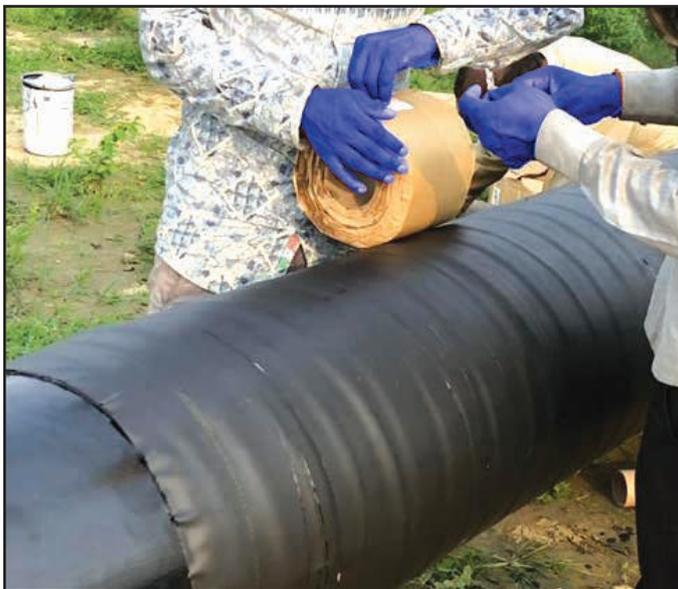
Densoclad 70HT™ Tape is spirally wrapped around the pipeline.
