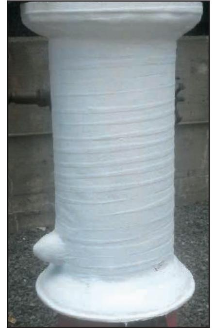
**Phase 1:** A coat of Archco™ 15 Acrylic Topcoat completes the 1<sup>st</sup> Denso system.
