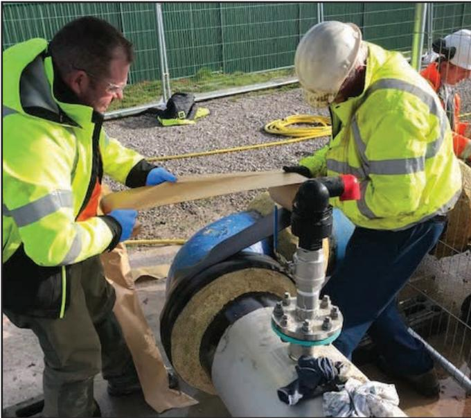
Above: Densoclad™ Tape is wrapped over Denso Profiling Mastic™ as part of the Denso P2 System™.
