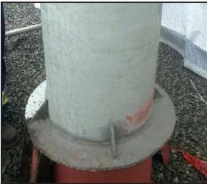
**Phase 1:** Spool piece cleaned and ready for the Denso™ 'Above Grade' system.
