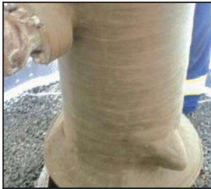
**Phase 1:** The application of Denso™ LT Tape over the Denso™ Paste.
