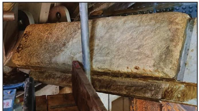
*A wrap of Denso™ Hi-Tack Tape completes the Steelcoat 100 System.*
