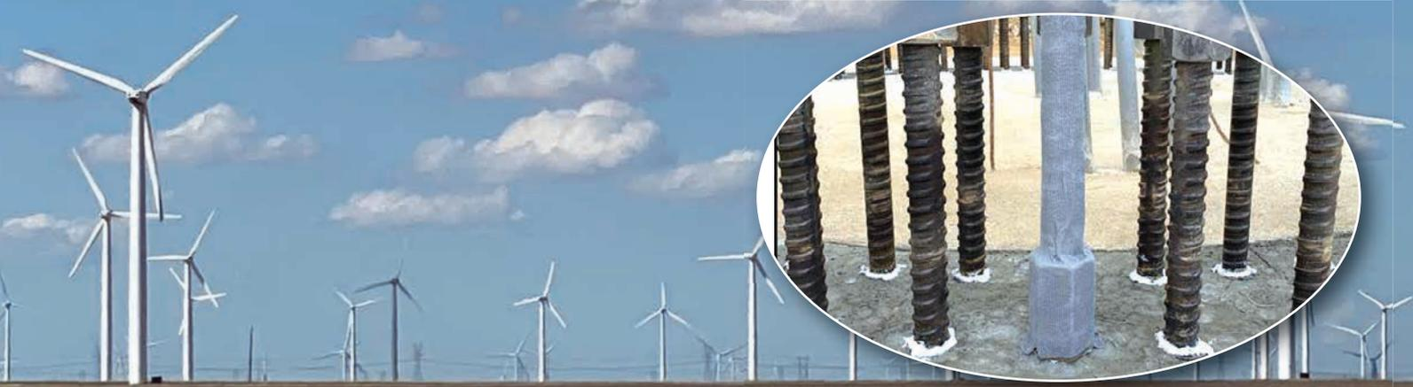
Over 900 wind turbine anchor bolts were protected from environmental corrosion with Denso™ ColorTape.
