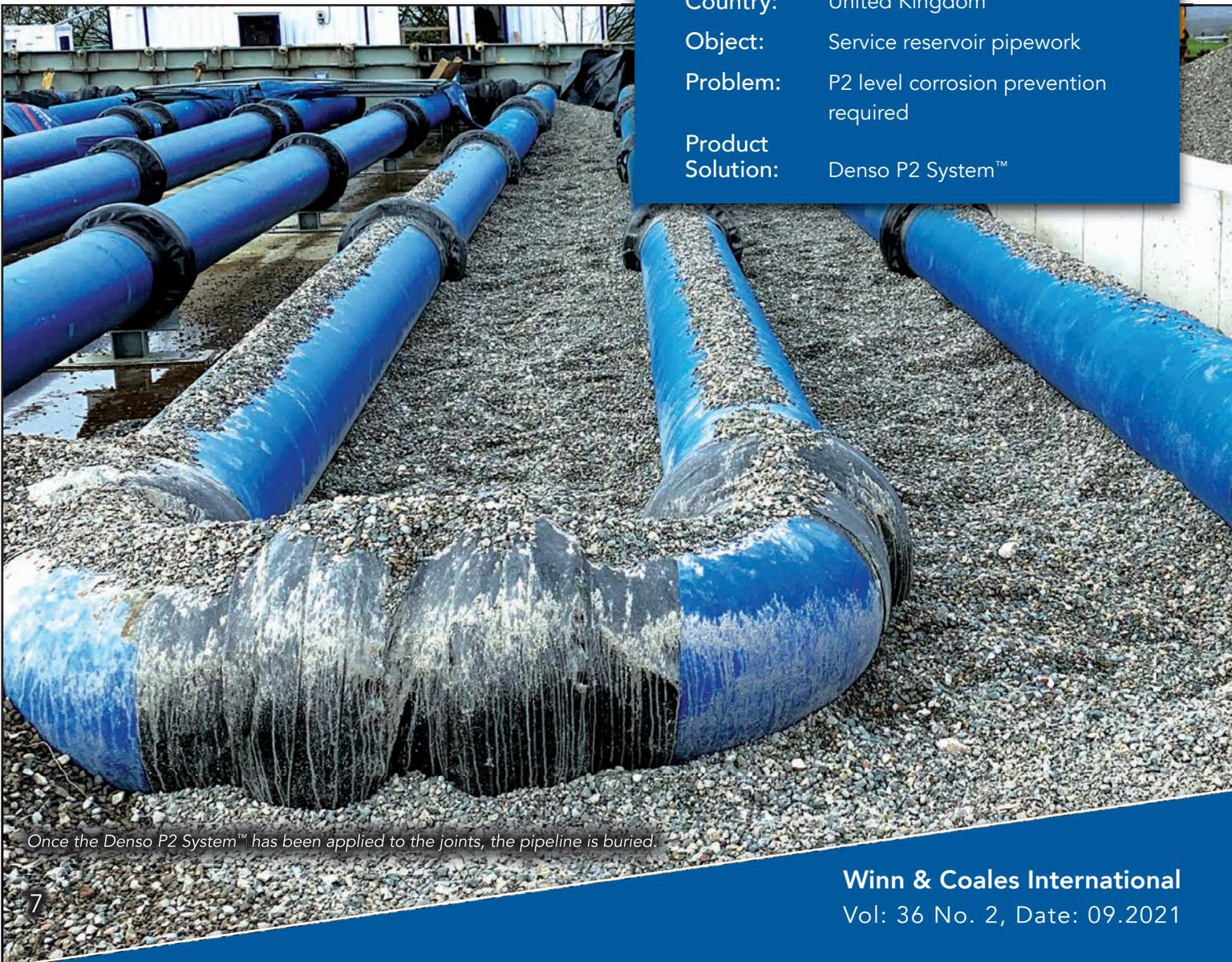
Once the Denso P2 System™ has been applied to the joints, the pipeline is buried.
