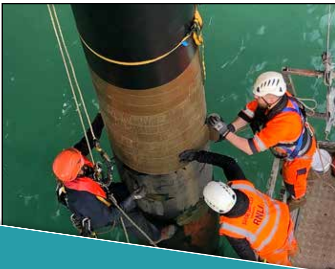
Denso™ Marine Piling Tape is wrapped around a pile.
