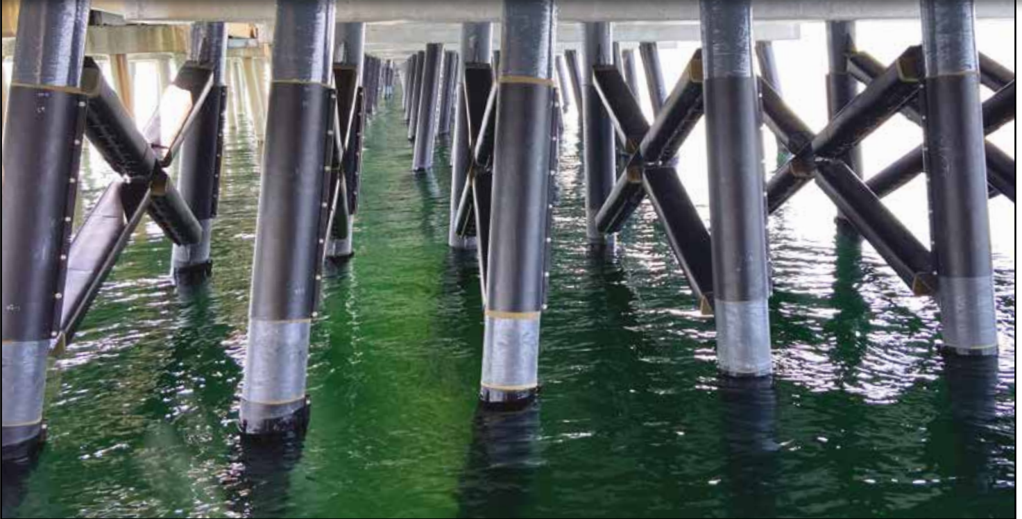
Above: Completed Cross-Bracing fully protected with the SeaShield Series 2000HD System as well as SeaShield 525 Epoxy at node areas.
