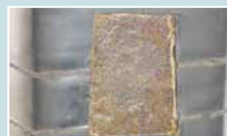
Outer layer panel removed to inspect the condition of pile surface.
