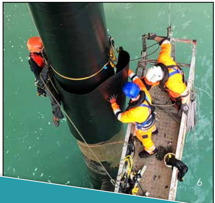
The outer HDPE jacket is wrapped around the pile.
