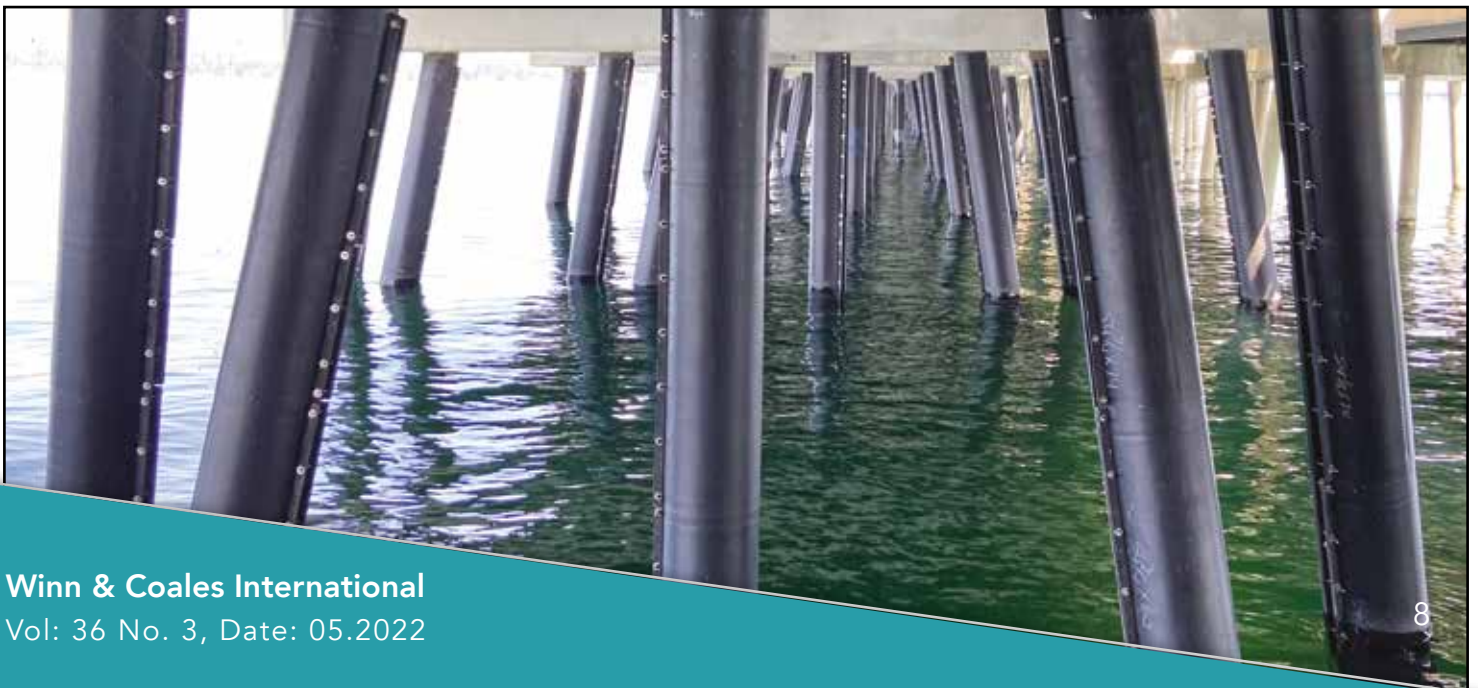
Completed 16" & 18" Dia. Cylindrical Piles fully protected with the SeaShield Series 2000HD System.
