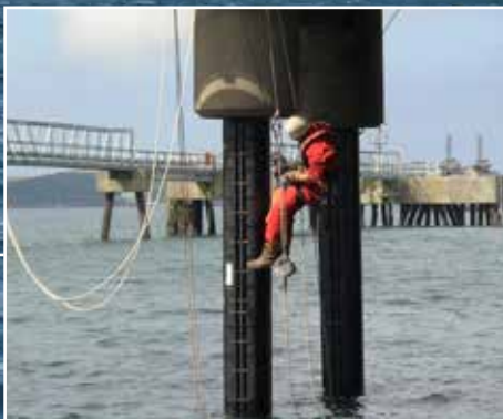
SeaShield System protecting loading jetty support piles - UK.
