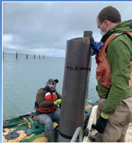
The SeaShield Fiber-Form™ System is applied to the wooden piles.
