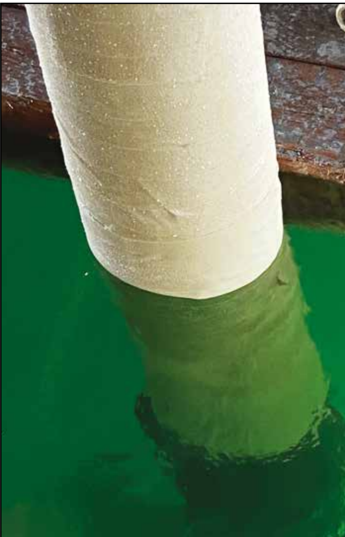
Above: Completed Cross-Bracing fully protected with the SeaShield Series 2000HD System as well as SeaShield 525 Epoxy at node areas.
