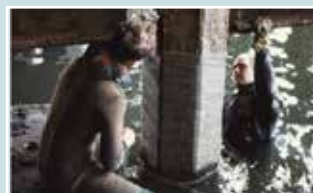
Underneath of jetty protected with a SeaShield Tape System.
