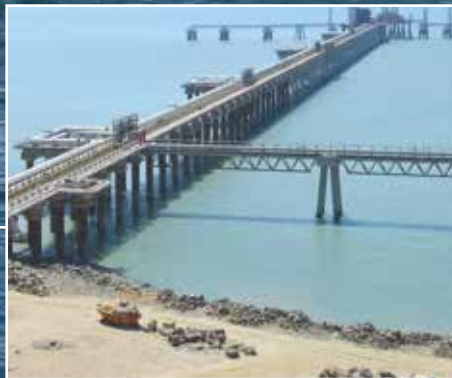
SeaShield System protecting LNG jetty support piles - India.
