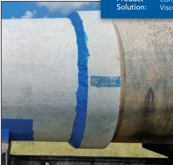
Above: Denso™ Glass Outerwrap coated with Denso™ Shield applied as the final mechanical layer.
