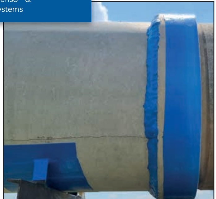
Below: Viscowrap™ ST applied with Viscomastic™ on concrete collar joint.
