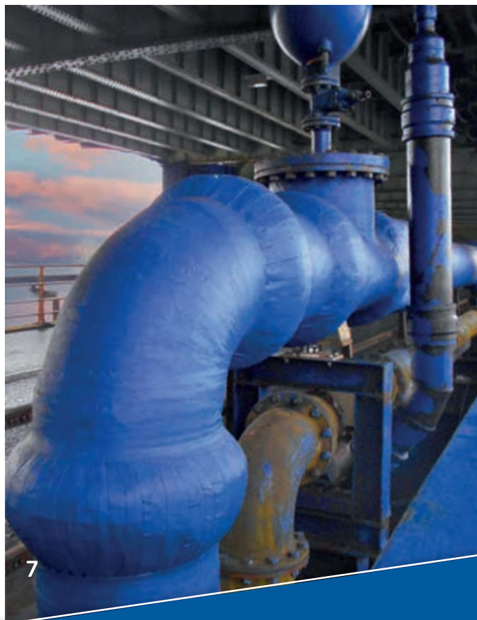
Above and below: The Denso™ Acrylic Topcoat that completes the Steelcoat 100/400 System protected waste water pumping main, was coloured blue to match the surrounding steelwork.
