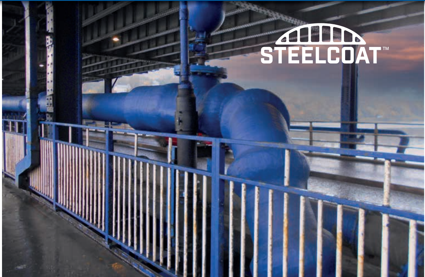
Above and below: The Denso™ Acrylic Topcoat that completes the Steelcoat 100/400 System protected waste water pumping main, was coloured blue to match the surrounding steelwork.
