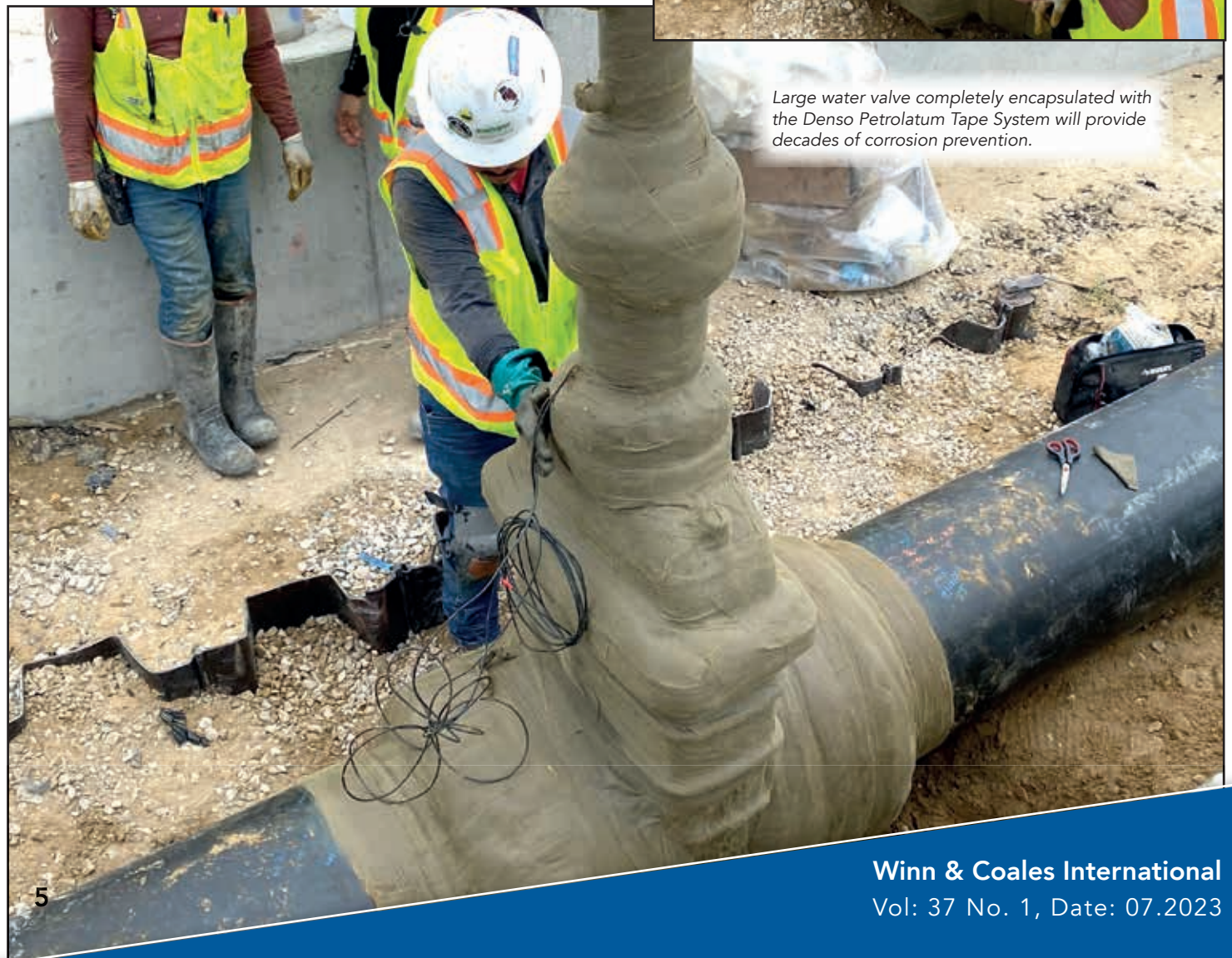
Opposite: A smooth profile is achieved with Denso Profiling Mastic prior to the application of Densyl Tape.
