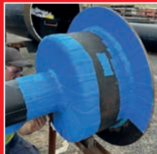
4. Viscowrap ST is applied.
