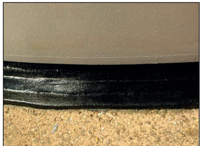
Applied Viscotaq™ EZ Wrapping with Denso™ Shield Topcoat.
