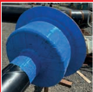
5. Complete Viscowrap ST wrap.
