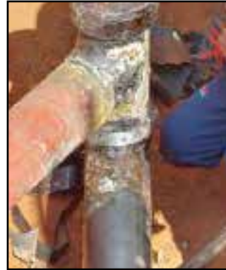
The surface condition once the existing shop applied coating was removed.
