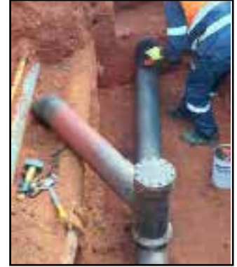
Denso Butyl P16HT™ Primer being applied in-situ by brush.
