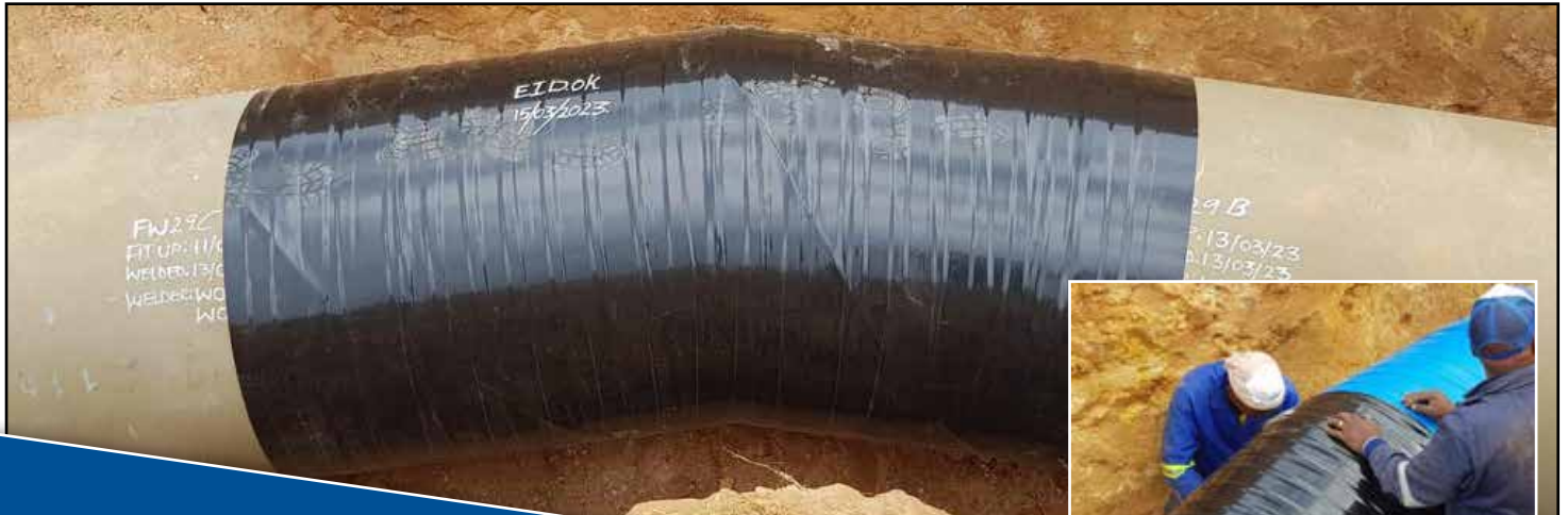
Denso™ PVC HD Self Adhesive Outerwrap being applied over the innerwrap.
