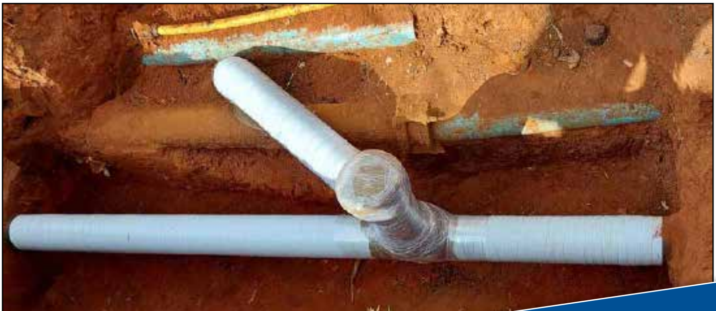
Denso™ Profiling Mastic and Denso™ Butyl Tape System applied to the prepared areas.
