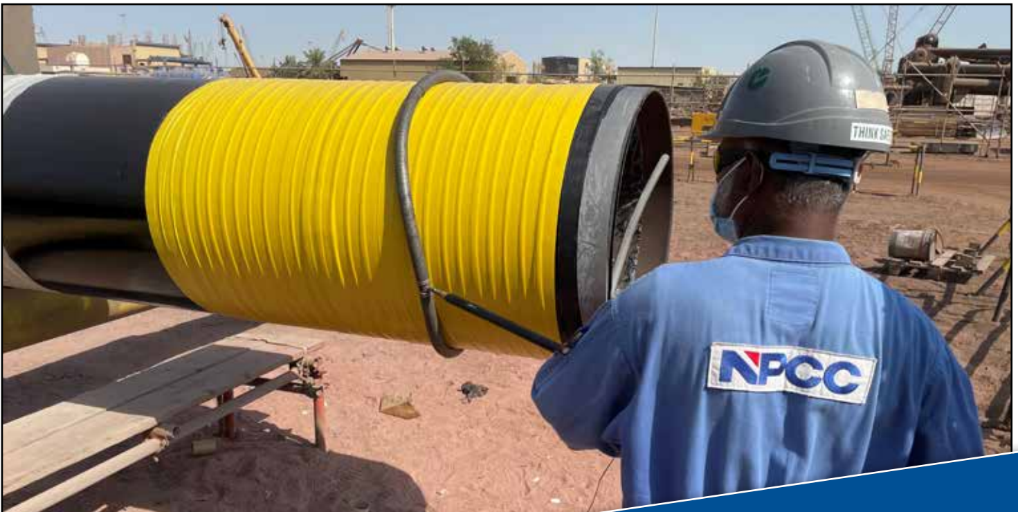
Denso PVC SA Tape™ is applied to the pipe lengths over the Densopol 80HT™, to give extra mechanical protection during transportation to the jobsite.
