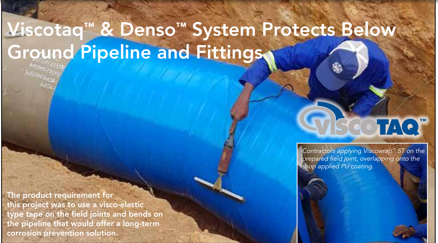
Above: Thorough holiday testing of the Viscowrap™ ST coating is carried out before the Denso™ PVC HD is applied.
