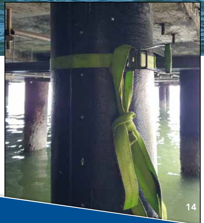
Below: Tensionable strapping is used to hold the SeaShield™ jackets in place during injection of the epoxy grout.
