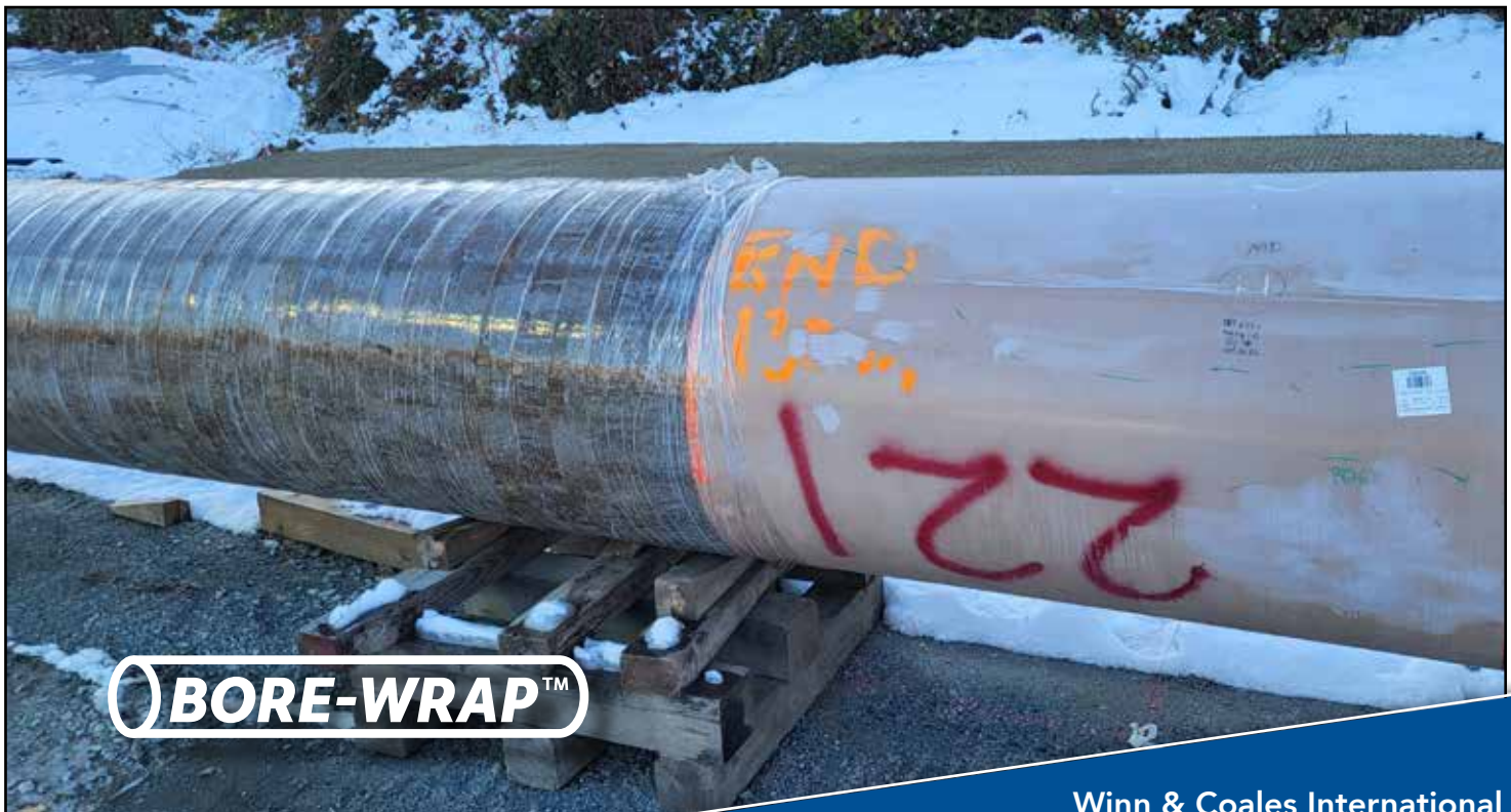
Denso Bore-Wrap™ application to wastewater pipeline
