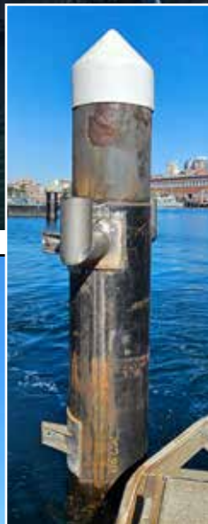
Inset: One of the piles with mooring hooks and brackets before application.
