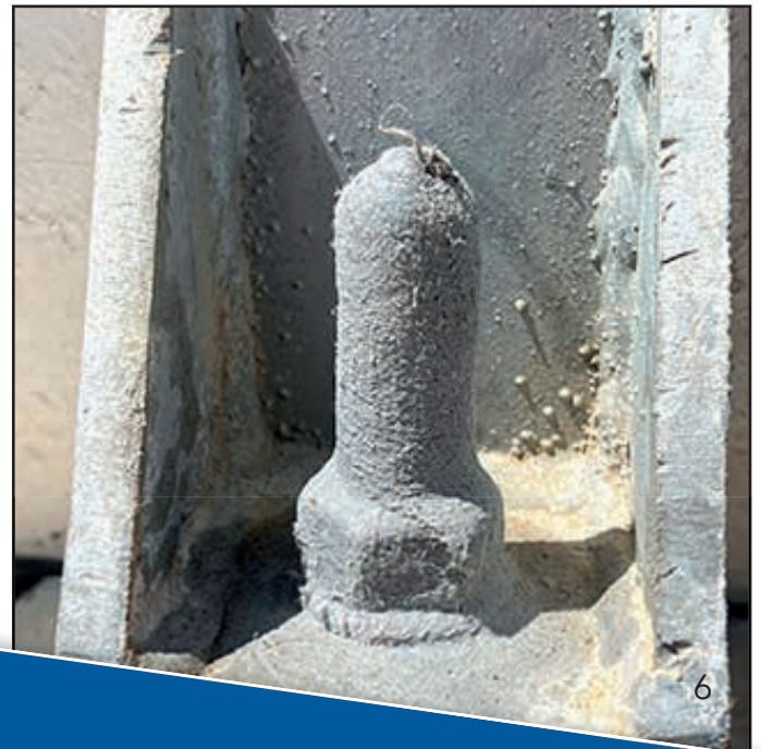
Steelcoat™ ColourTape applied to M20 threaded rounded bars/nuts.
