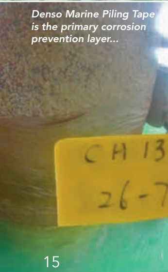
...This is followed by a HDPE Jacket in both systems.
