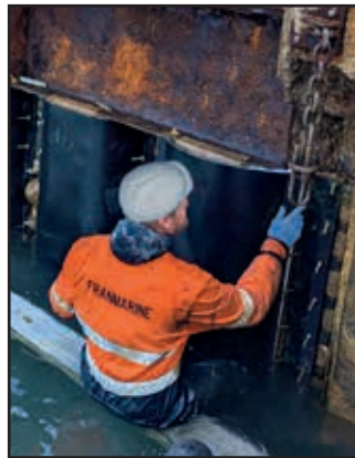
Installation of HDPE Jackets.
