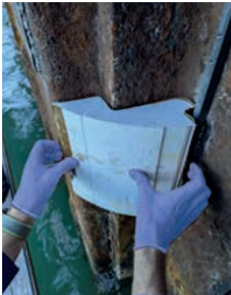
Application of Foam Filler.
