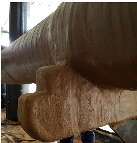
Before and after application of the Denso Petrolatum Tape System.
